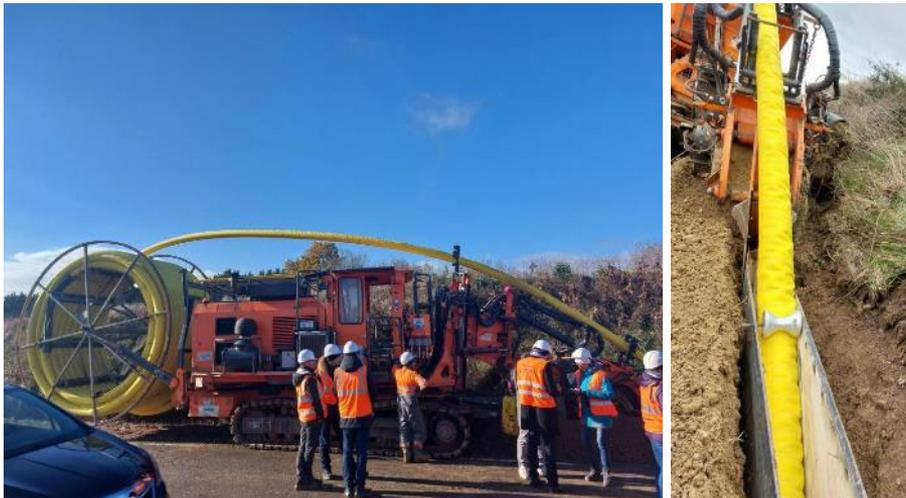
The recently acquired Gaillon plant (DYKA France) is now producing PE pipes with a new, innovative wrapping technique aimed at reducing the environmental impact of gas pipe-laying sites.
