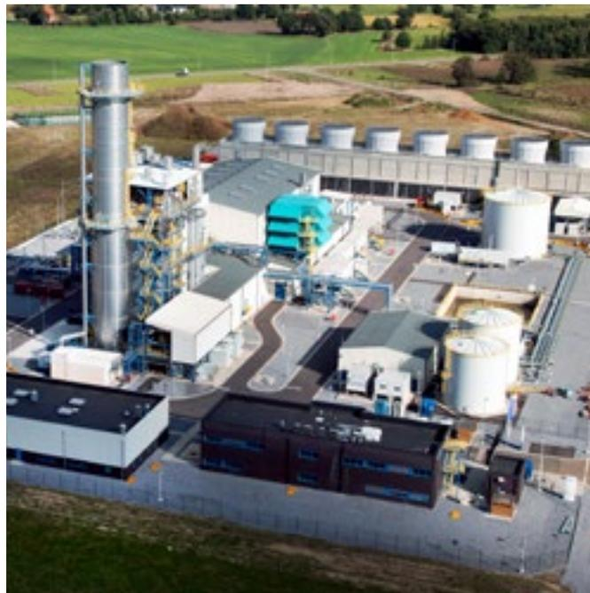
The **T-Power** segment includes the activities of Tessenderlo Group regarding the generation of electricity, in particular, the 425 MW CCGT power plant (Combined Cycle Gas Turbine) of T-Power.
