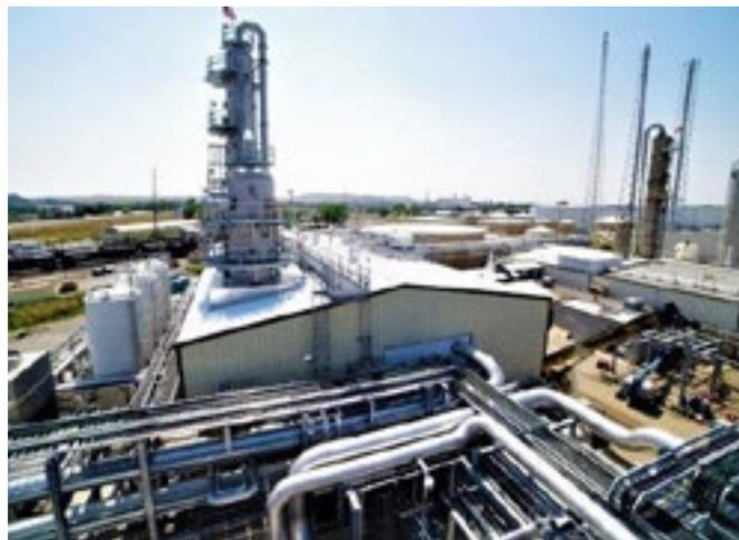
At **Tessenderlo Kerley, Inc.** we provide sulfur recovery processing for several refineries where our facilities reduce the incoming  $H_2S$  content of the gas by 99.9985% before venting to the atmosphere. The environmental performance of our facilities remains well below the typical US EPA permit limits that have been set for  $SO_2$  emissions.
